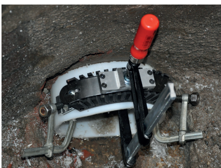
Anchoring the pipe to a concrete wall such as a manhole.
