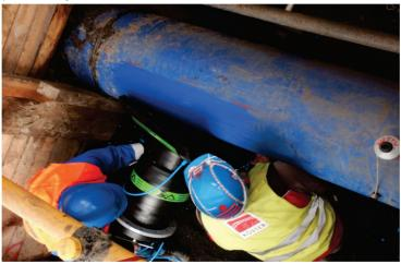
The solution and economical alternative to a spigot Tee for integrating a branch line under operating pressure was provided by the spigot saddle FRIALEN SA XL characterised by:
