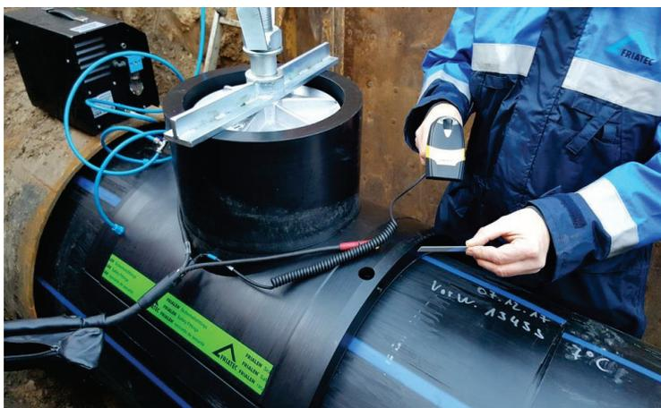
The time frame for the installation was extremely short, just three months from October to December, putting the contractor under huge pressure. Yet this challenge could be met successfully with the FRIALEN spigot saddles SA XL d 710 with d 400 outlet and a number of large couplers XL UB d 710 and d 800. The interaction of these components with the preconfigured equipment worked yet again.
