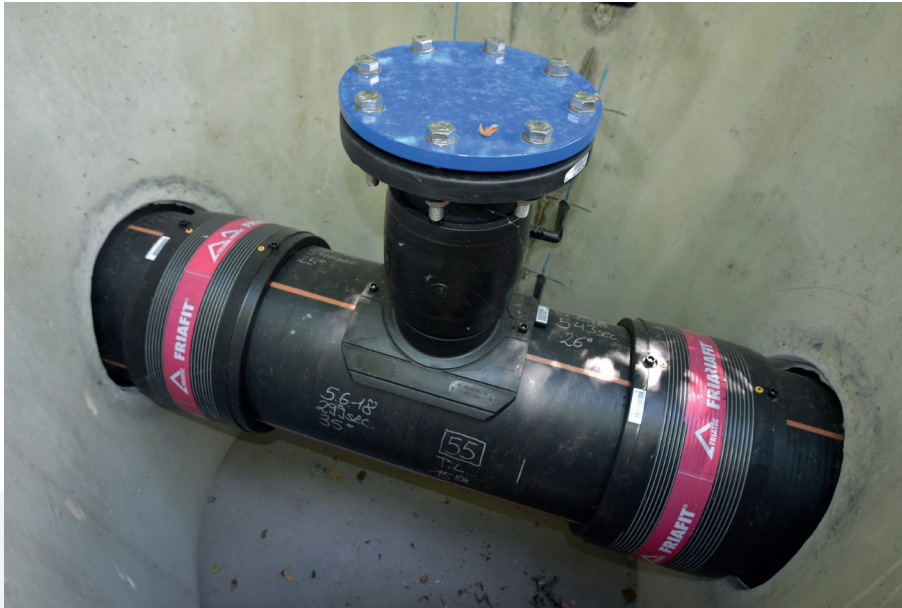
Flanged access covers are provided in the manhole for later inspections
