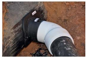
Fig 5 – Connection with sewage saddle ASA TL and bend ABMS
