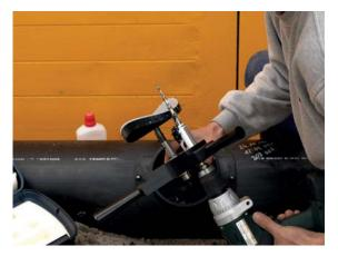
Fig 3b - Pipe cutout being removed
