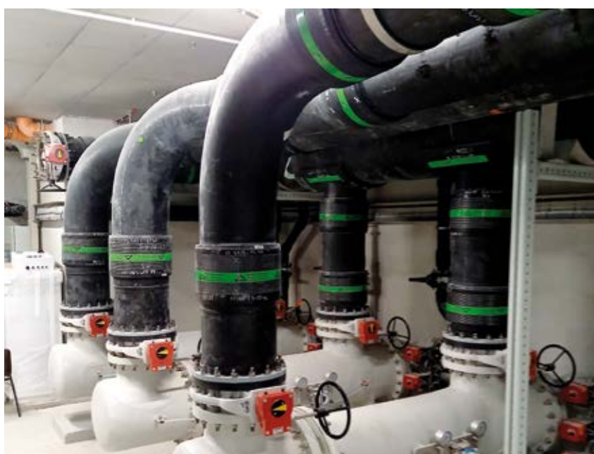
The new PE pipelines in the pumping station
