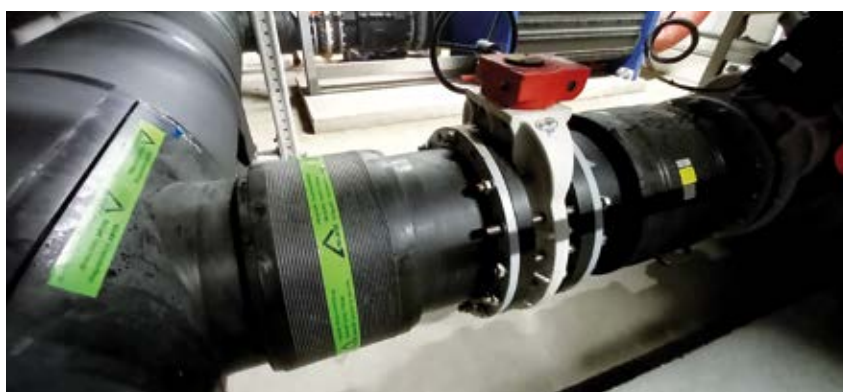
Branching using saddle SA XL, coupler UB and valve FK
