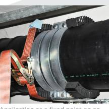
Application as a fixed point on an overhead pipeline.
