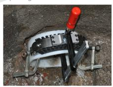
Anchoring the pipe to a concrete wall such as a manhole.
