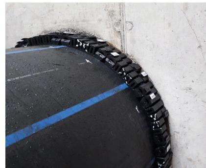
**Strength per fixed point 40 kN, when using several FIXBLOCs on the pipe, higher forces can also be absorbed.**
