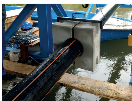
Use as a fixing for sink weights for under water pipelines.
