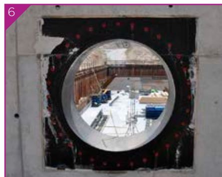
Clean the sealing surface and remove the plugs
