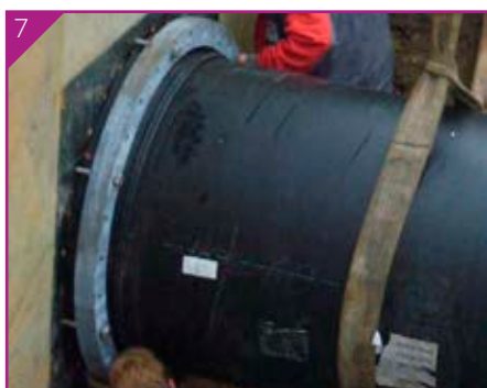
Fitting the connecting line
