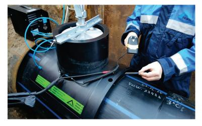
The time frame for the installation was extremely short, just three months from October to December, putting the contractor under huge pressure. Yet this challenge could be met successfully with the FRIALEN spigot saddles SA XL d 710 with d 400 outlet and a number of large couplers XL UB d 710 and d 800. The interaction of these components with the preconfigured equipment worked yet again.
